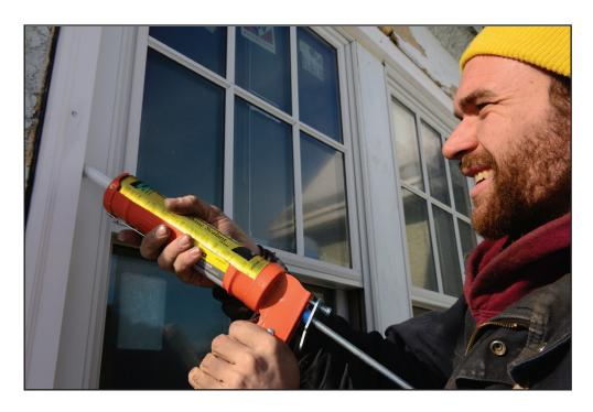
stream, and make sure it sticks to both sides of the crack or seam. Afterwards, use a putty knife to smooth out the caulk, then wipe the surface with a dry cloth.
